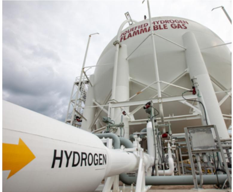
Figure 4: 20 m diameter LH<sub>2</sub> storage tank in NASA Kennedy Space Centre, Courtesy of NASA
